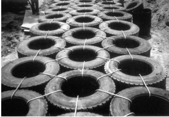
FIGURE 1.12 Truck tires used for crash barriers. 1
