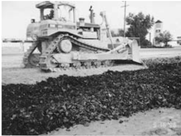
FIGURE 1.14 Tire chips for a roadbed application. 1
