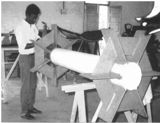
Figure 3.2 Rubber lining of gypsum agitator for a fertiliser factory
